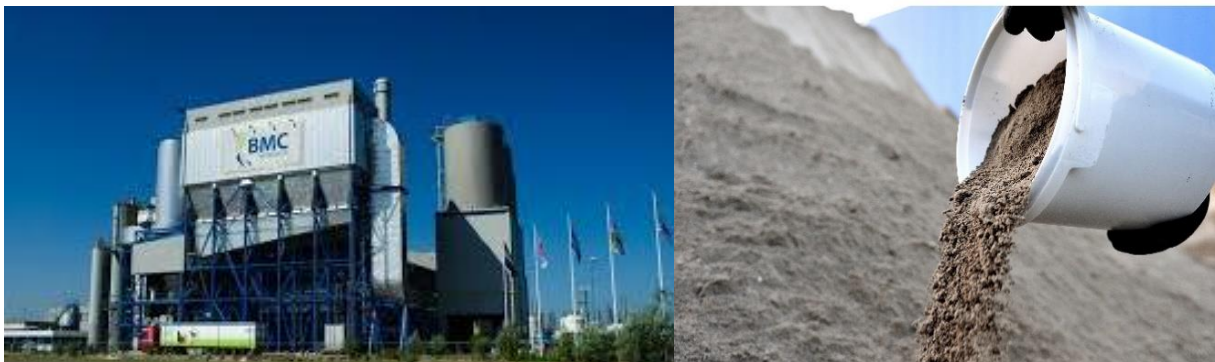
Figure 3.1. Pictures of the production plant of poultry litter ash (PLA) of BMC in Moerdijk (left) and close up of the end product, PLA (right).
