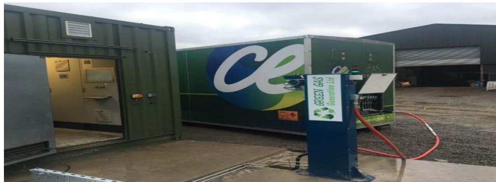
Figure 3: Biogas transporting trailer with filling station on the Nurney site.
