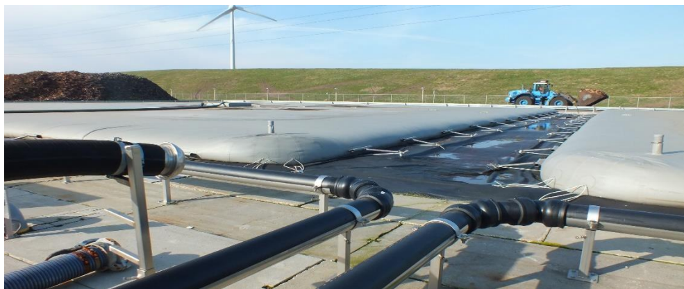
Figure 3: Storage bag tanks for Ammonium sulphate.
